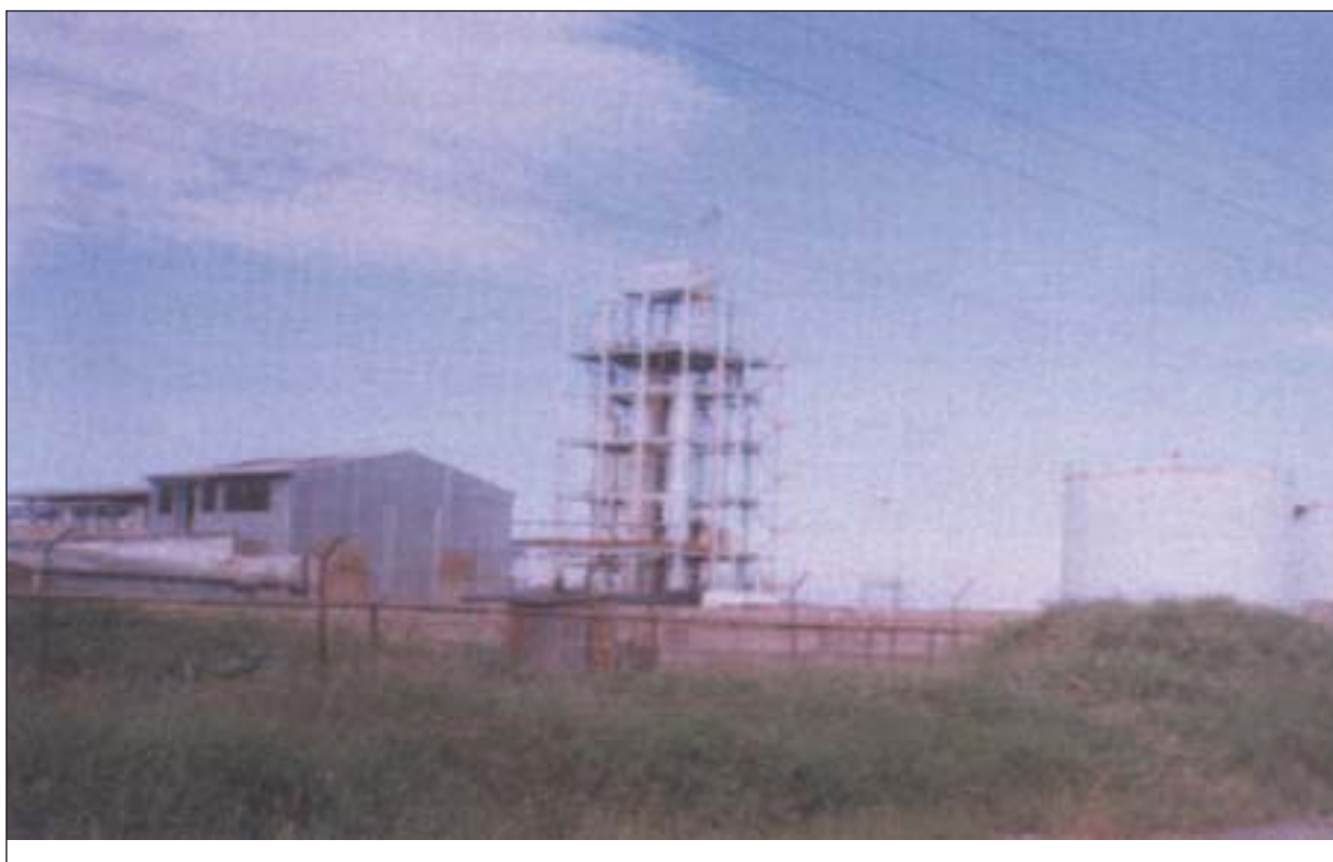
Figure 2.1: Ethanol Plant at Dwangwa, Malawi
