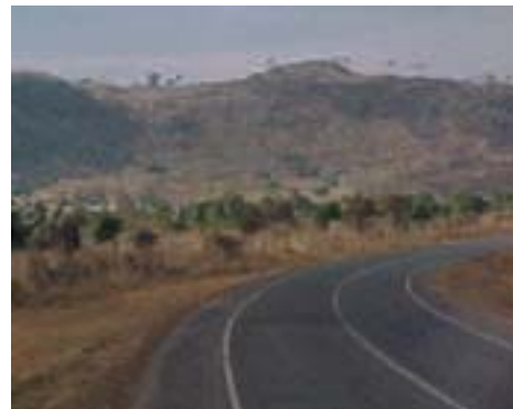
Figure 1.9 (b): Bituminised road.
